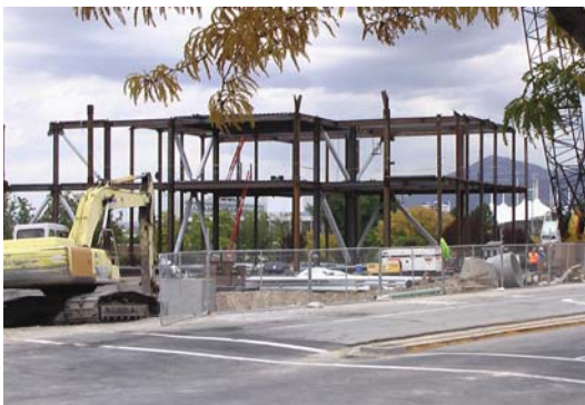
Hinckley Alumni Building during construction (white members are buckling-restrained braces)
