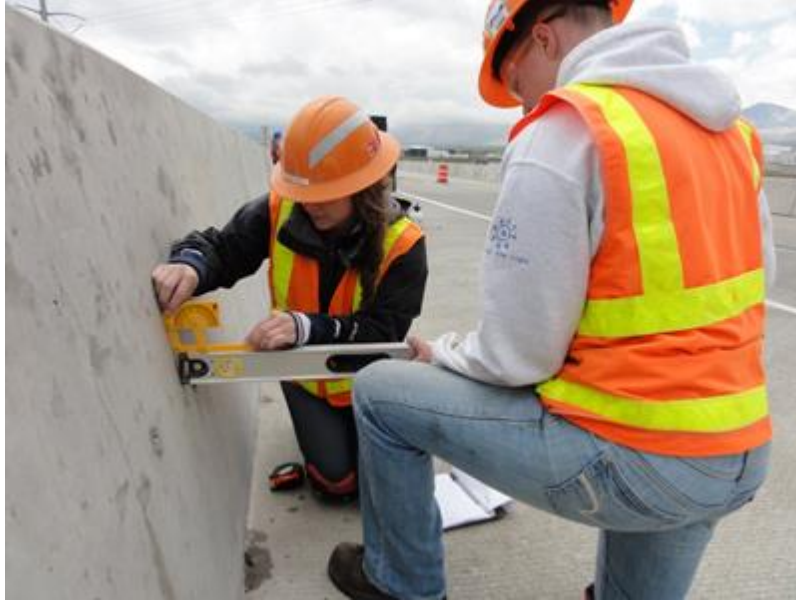
Figure 3.4 Measurement of a wall angle.
