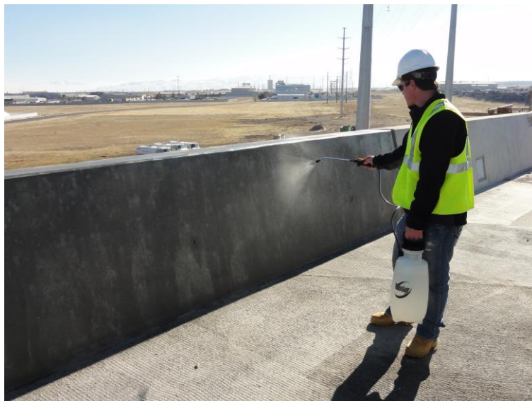
Figure 3.7 Application of sealant to a concrete wall.
