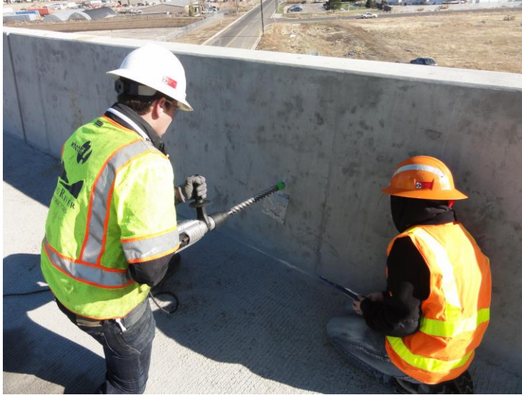
Figure 3.5 Drilling of a concrete wall.
