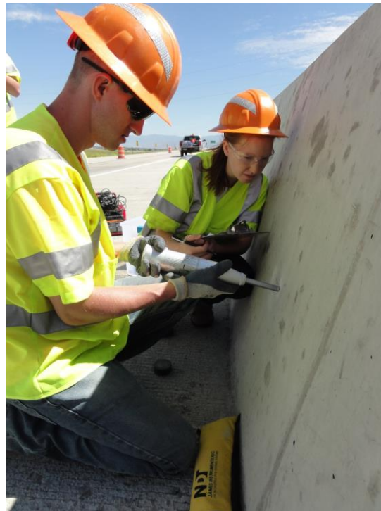
Figure 3.3 Schmidt hammer testing.
